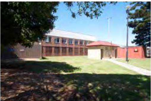
14 Victoria Road Wicks Park
